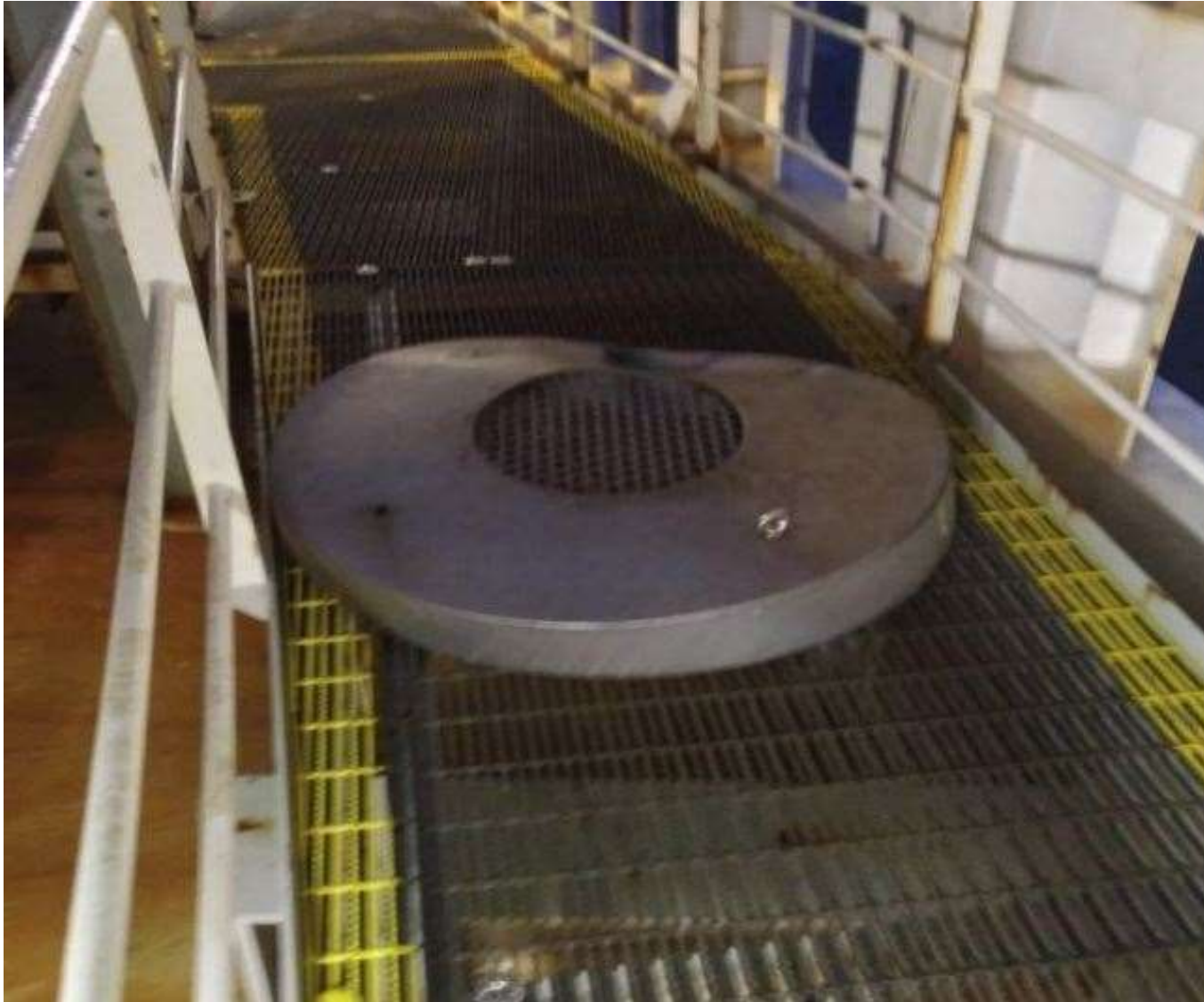
Figure 2: Lid after it had fallen down on walkway
